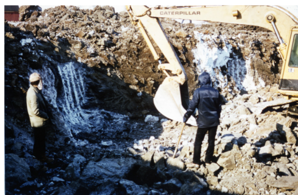
Fig. 7 Great ice-wedges in a foundation cavity on road 232. Normally traceable by ground inspection. Photo O. Gregersen
