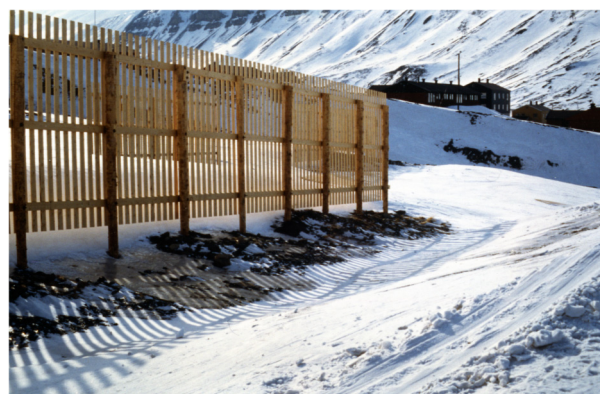
Fig.11 Snow fence before strengthening the construction and adjusting the ground clearance. Photo E. Hestnes
